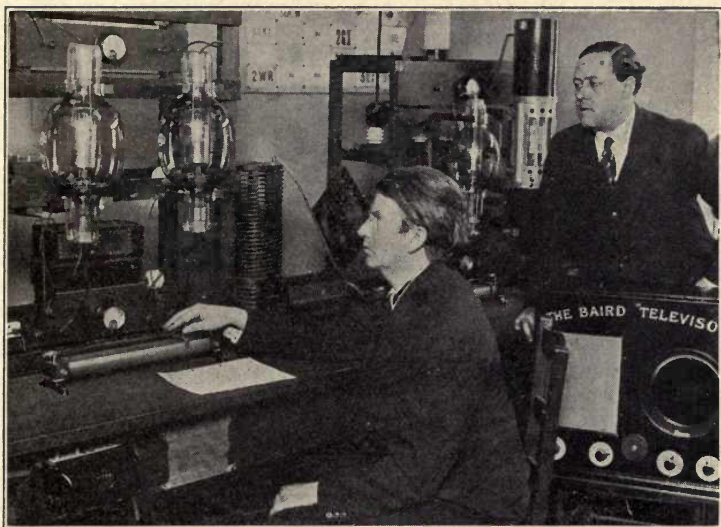
FIG. 79.—A close-up of the first transmitter used in trans-Atlantic television tests.
